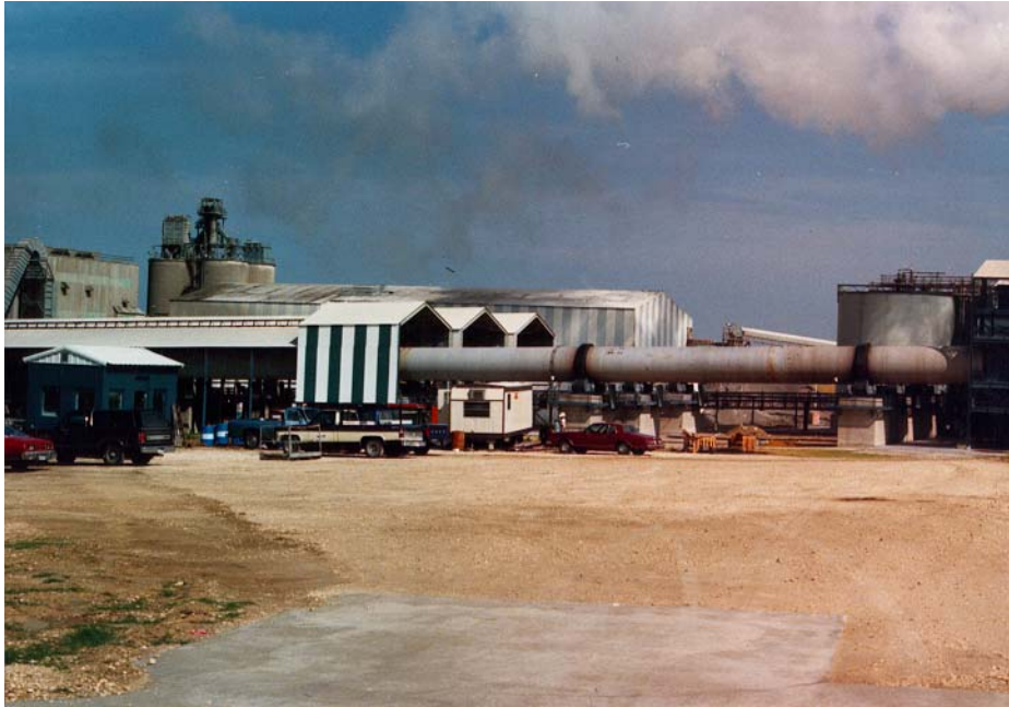
The Gilford Hill Cement Plant located in Dallas, Texas. Kiln manufactured by Ford Bacon & Davis.
